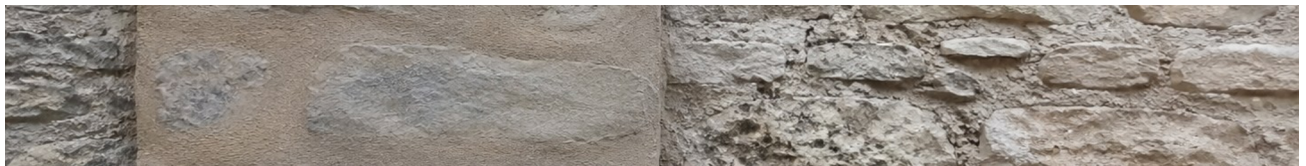
Photograph 3. The panel is approved dry. A wet mix tells you nothing about the finished colour or texture.
