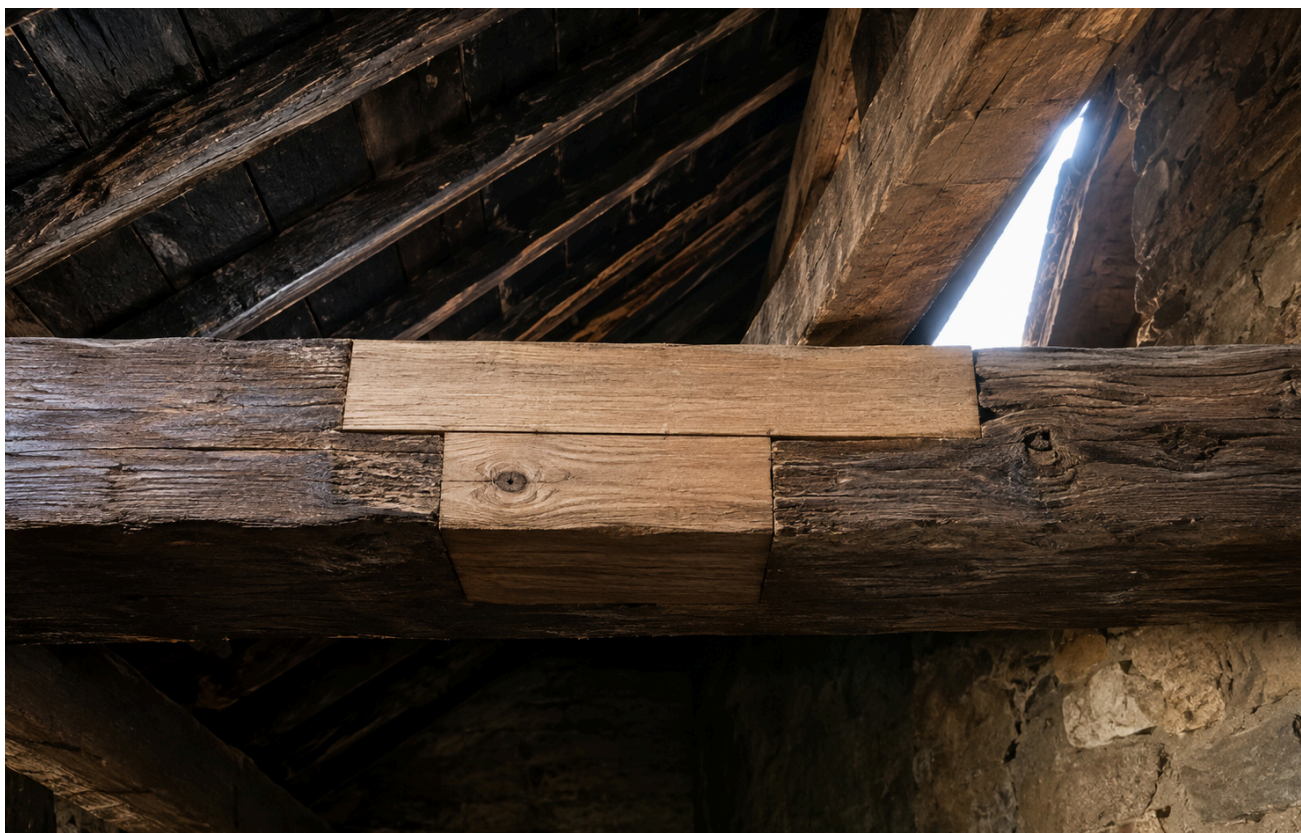
Photograph 6. Rung four of the ladder. The decayed section has gone and everything sound around it has stayed.
