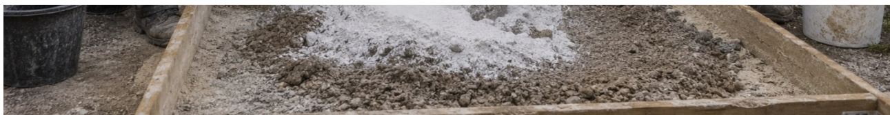
Photograph 4. Quicklime and damp aggregate, gauged and ready to be turned. The reaction is exothermic and vigorous, and it is done in full protective equipment.
