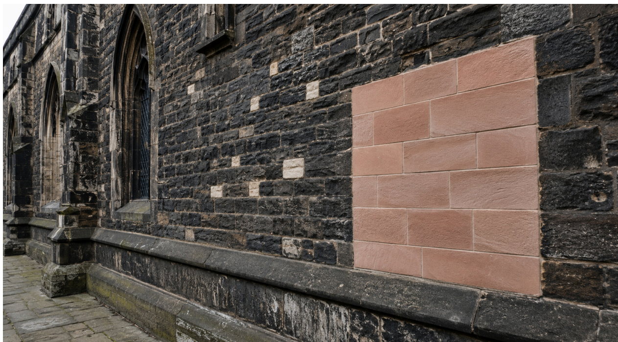
Photograph 7. Two approaches on one elevation. The indents read as repair; the replaced panel reads as a scar and will for a century.
